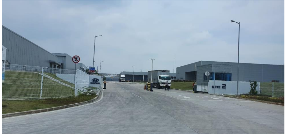
Photo of Hyundai industrial estate
